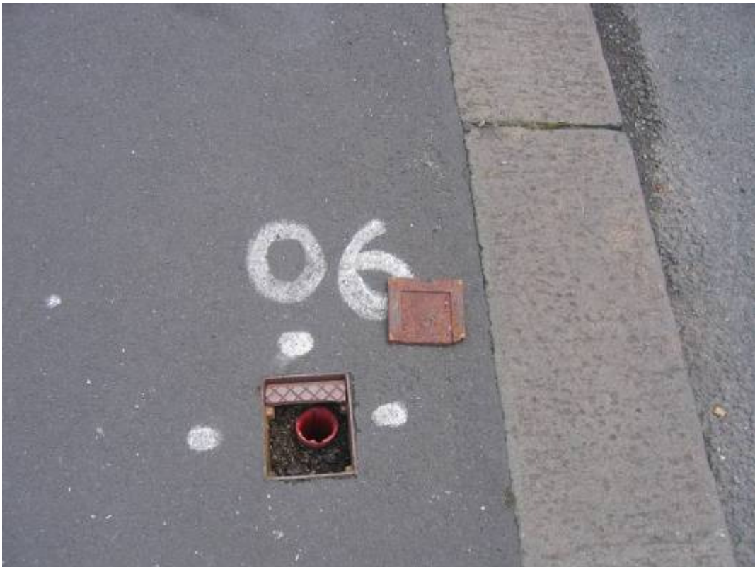
Plate 29 Scarborough South Cliff D1 (AA06)
