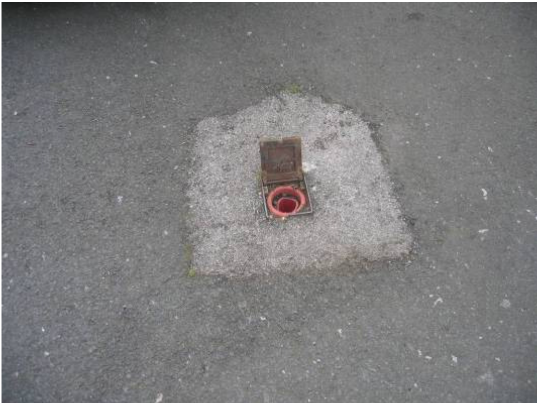
Plate 6 Scarborough North Bay L11
